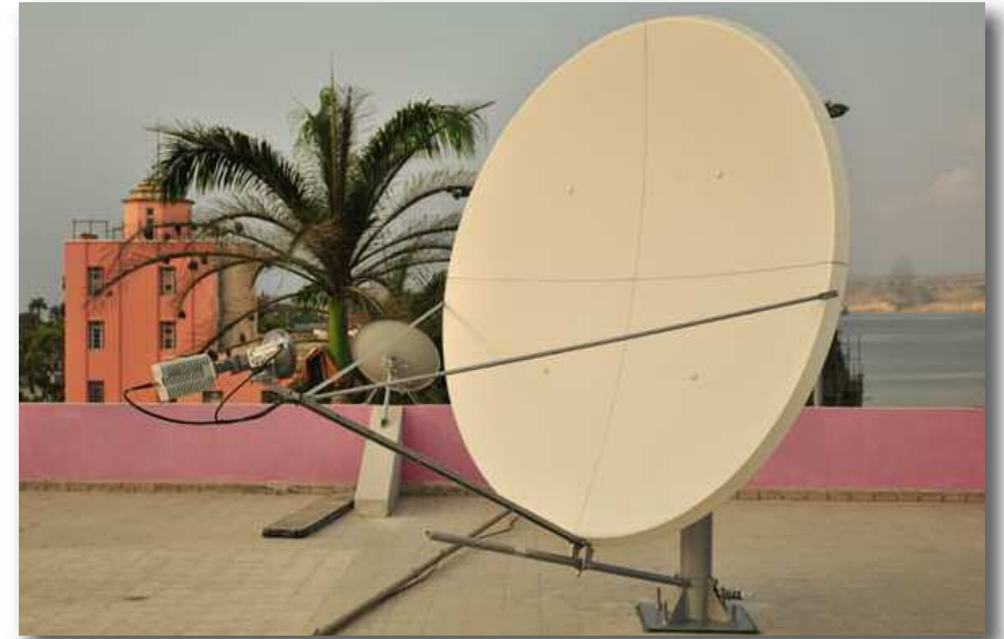
BusinessCom C-Band Remote VSAT Equipment ODU (Outdoor Unit) with Prodelin 1383 Antenna
