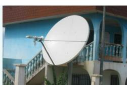
2.4m iDirect Infiniti VSAT on NSS-7
